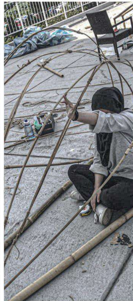
SLAT SPLINE STRUCTURE
