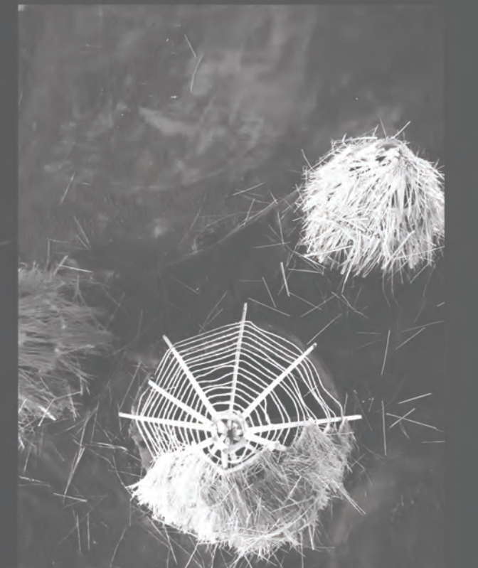
FILLING BAMBOO RAFTERS
