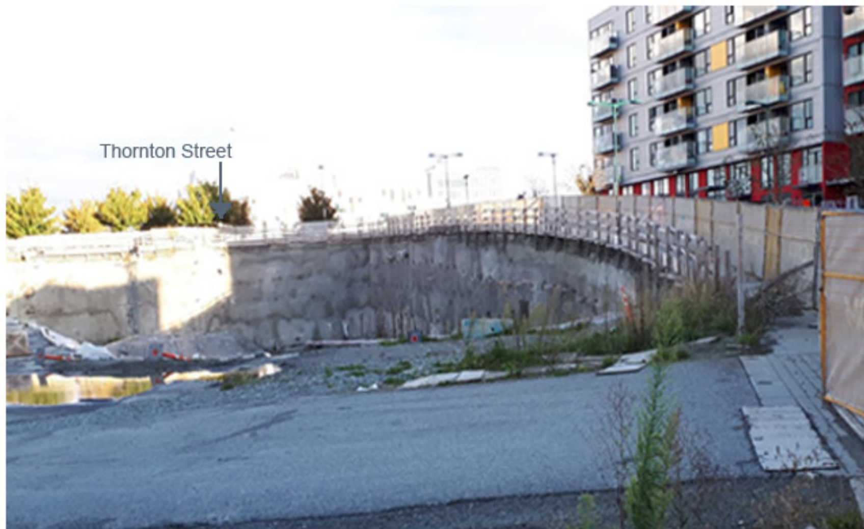
Photo of the site looking from east direction to west
